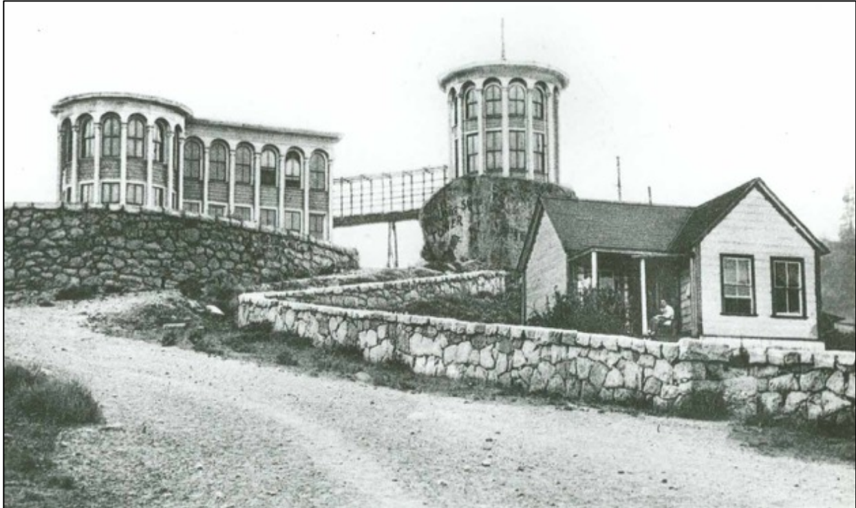
Figure 2. 1906 McGlashan's 'Crystal Palace' and Law Office; note retaining wall (HIGH007)
